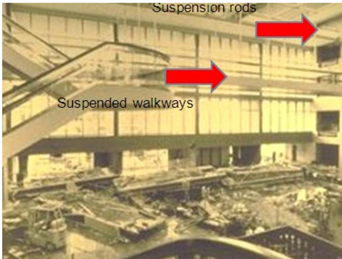
Figure 5 Suspended Walkways at the Atrium Lobby
